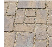
Figure 31 Permeable pavers applied to the turning radius
